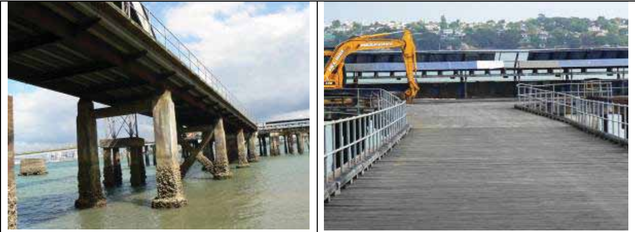
Chelsea Wharf – reinforced concrete pillars, steel substructure with wooden decking.
