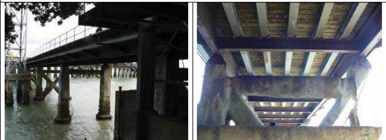
Chelsea Wharf – chlorinated rubber coated and Gold Seal over-coated steel substructure.
